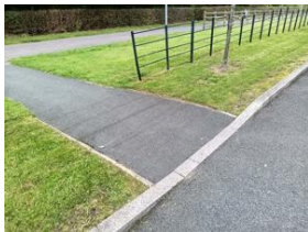
Image Notes: Spraying of kerbs and grass cutting.
