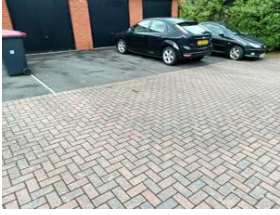
Image Notes: Courtyard maintenance
