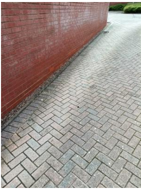
Image Notes: Courtyard maintenance
