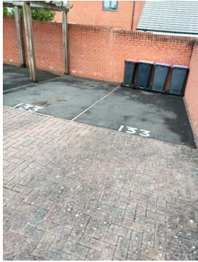
Image Notes: Courtyard maintenance
