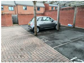
Image Notes: Courtyard maintenance
