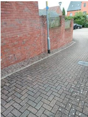
Image Notes: Courtyard maintenance
