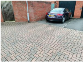
Image Notes: Courtyard maintenance
