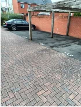
Image Notes: Courtyard maintenance
