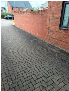
Image Notes: Courtyard maintenance
