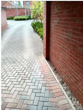
Image Notes: Courtyard maintenance
