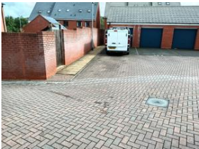
Image Notes: Courtyard maintenance
