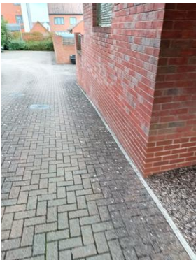
Image Notes: Courtyard maintenance
