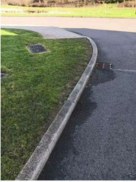
Image Notes: Cleaning and edging kerbs
