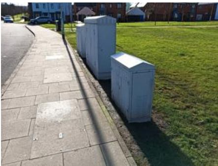
Image Notes: Cleaning and edging kerbs
