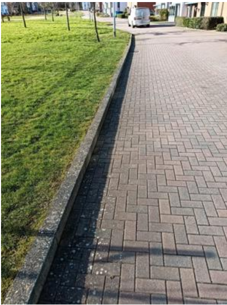
Image Notes: Cleaning and edging kerbs
