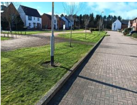
Image Notes: Cleaning and edging kerbs
