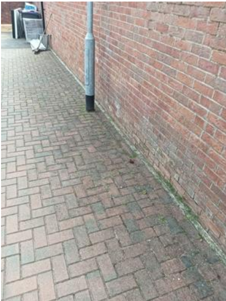
Image Notes: Courtyards maintained and sprayed
