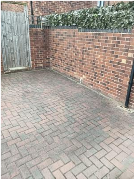
Image Notes: Courtyards maintained and sprayed
