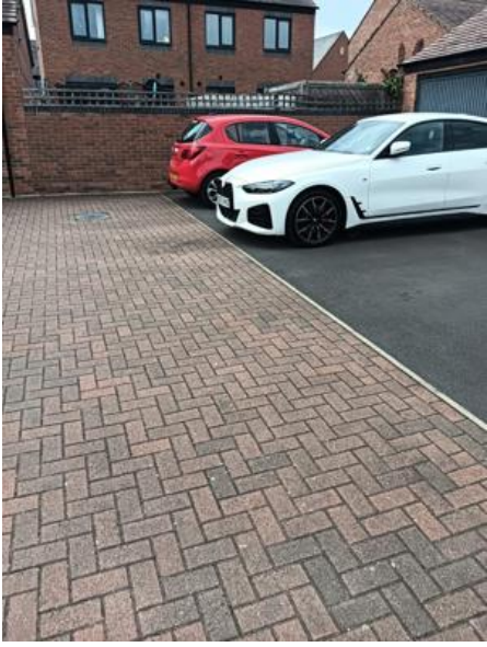
Image Notes: Courtyards maintained and sprayed
