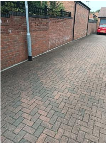
Image Notes: Courtyards maintained and sprayed
