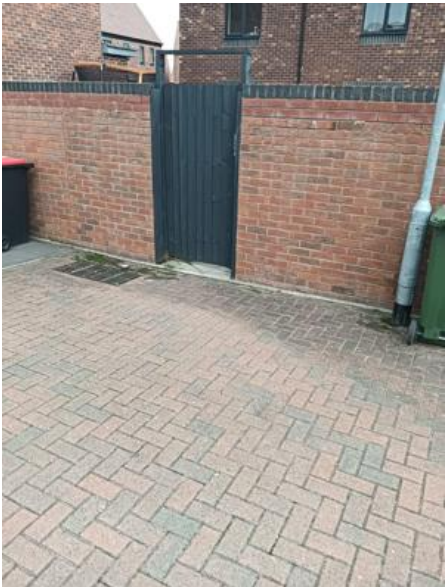
Image Notes: Courtyards maintained and sprayed
