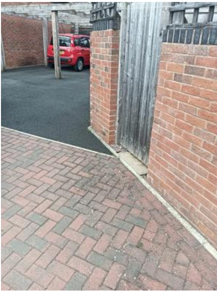
Image Notes: Courtyards maintained and sprayed
