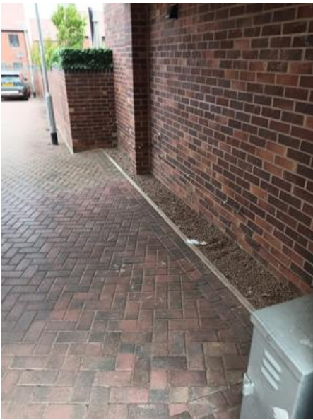
Image Notes: Courtyards maintained and sprayed
