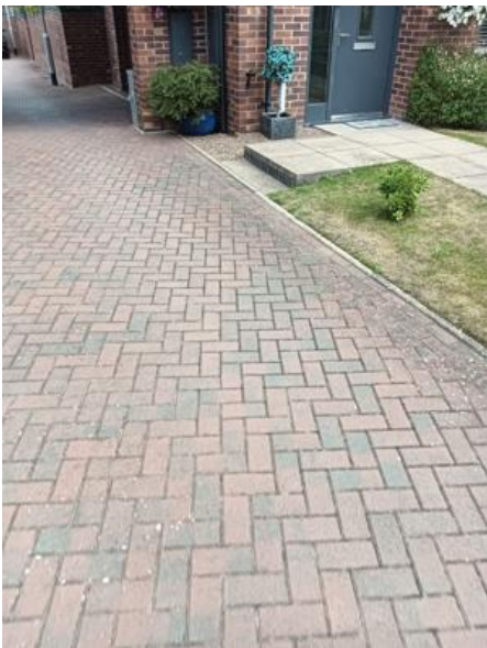
Image Notes: Courtyards maintained and sprayed
