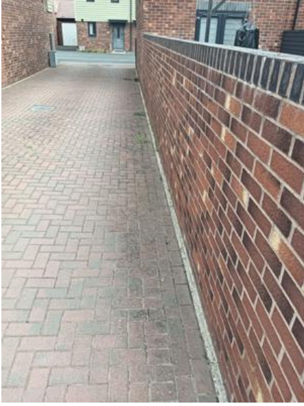
Image Notes: Courtyards maintained and sprayed
