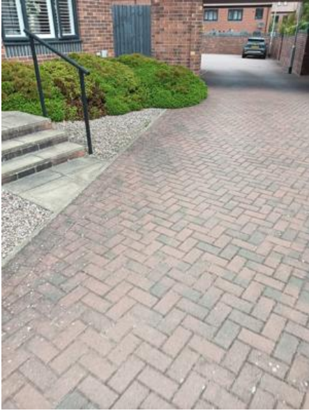
Image Notes: Courtyards maintained and sprayed
