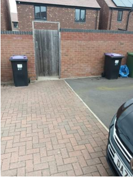
Image Notes: Courtyards maintained and sprayed
