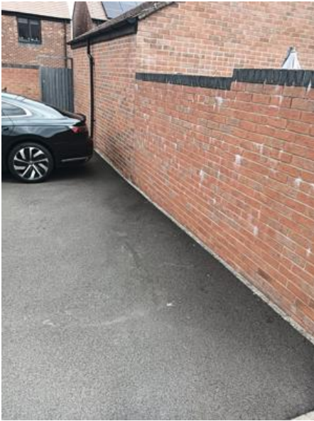
Image Notes: Courtyards maintained and sprayed
