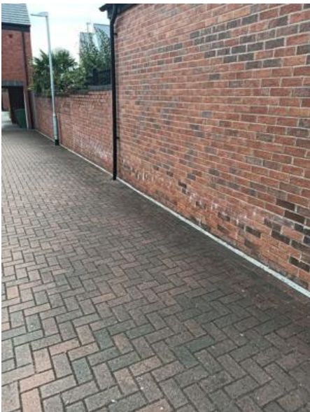
Image Notes: Courtyards maintained and sprayed
