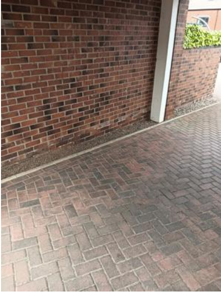
Image Notes: Courtyards maintained and sprayed
