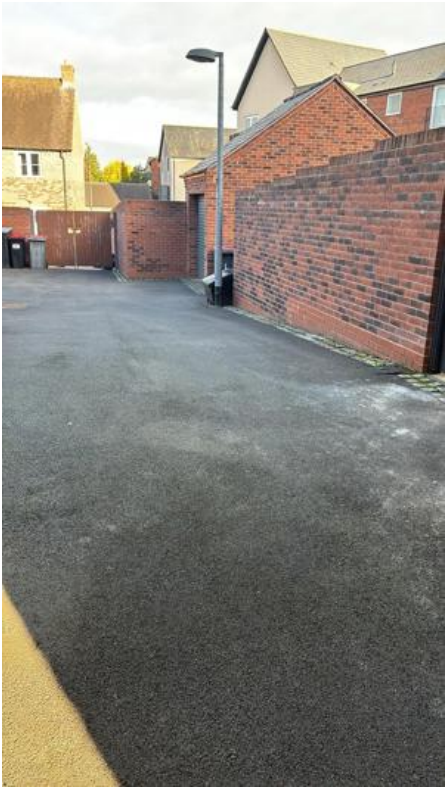
Image Notes: Courtyards blown and sprayed.
