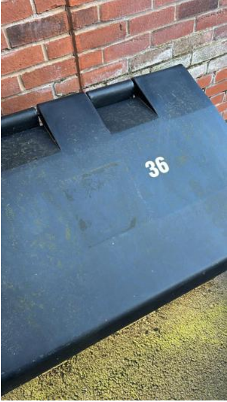
Image Notes: Courtyards blown and sprayed.
