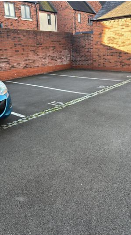
Image Notes: Courtyards blown and sprayed.
