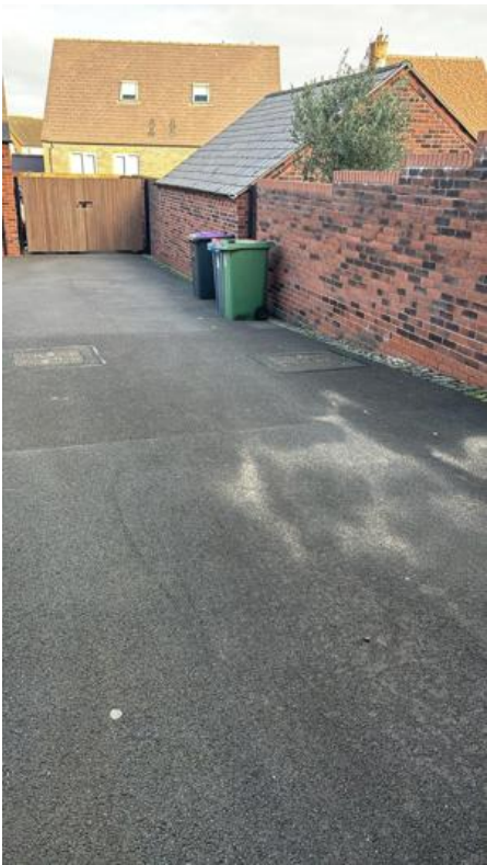
Image Notes: Courtyards blown and sprayed.
