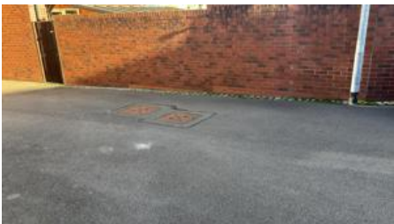
Image Notes: Courtyards blown and sprayed.
