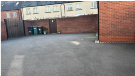
Image Notes: Courtyards blown and sprayed.
