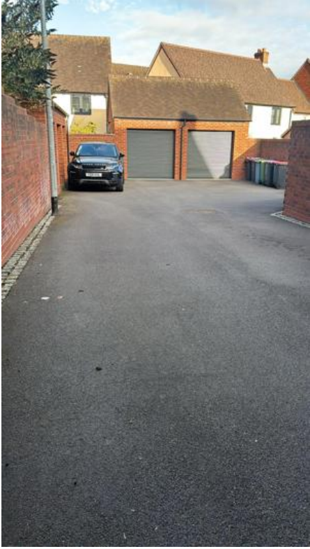
Image Notes: Courtyards blown and sprayed.
