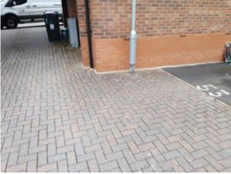
Image Notes: Courtyard sprayed
