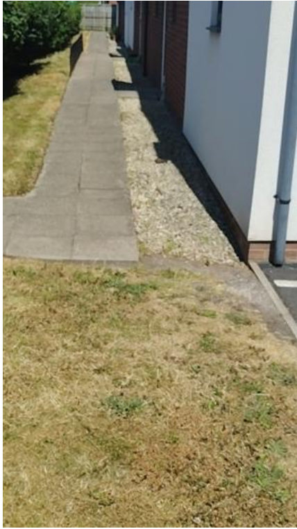
Image Notes: Outside flats sprayed.
