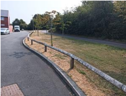
Image Notes: Kerb sprayed grass cut
