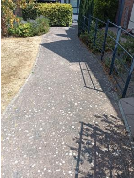
Image Notes: Paths sprayed and kerbs
