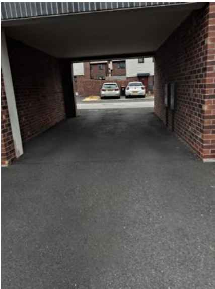
Image Notes: Courtyard sprayed
