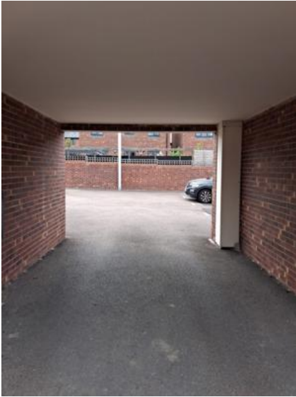
Image Notes: Courtyard sprayed
