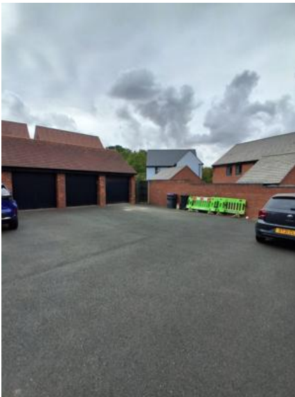
Image Notes: Courtyard sprayed
