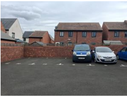
Image Notes: Courtyard sprayed
