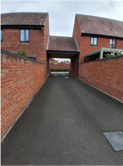
Image Notes: Courtyard sprayed
